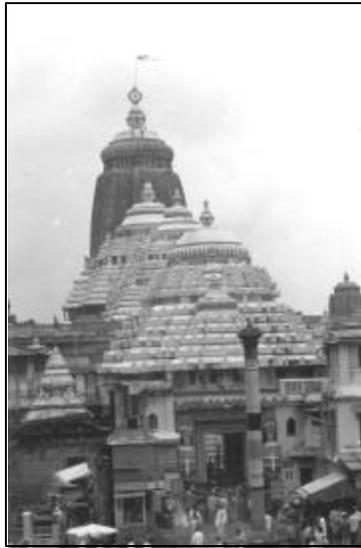
Subsequently cracks were noticed by Archaeological Survey of India in different portions of the main temple. In order to ascertain the actual cause, it was felt necessary to deplaster the whole lime plaster and accordingly the job was entrusted to an expert committee to study the conservation
